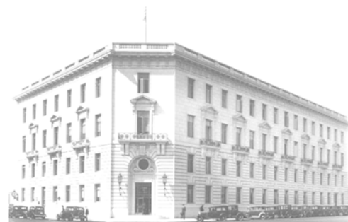
San Francisco Department of Public Health at 101 Grove Street (1935)
